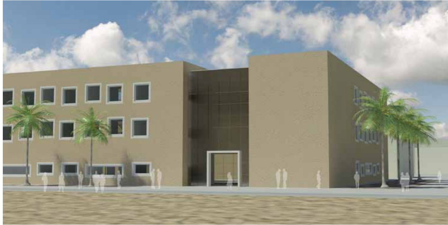
Daylight perspective of the main entrance
